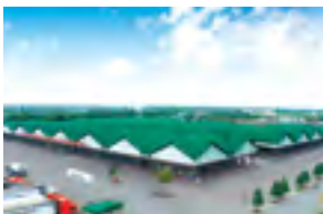
Thuduc Agriculture Wholesale Market (Thu Duc District) (TDH: 100%) Land area: 200,000 m 2 Completed in 2003
