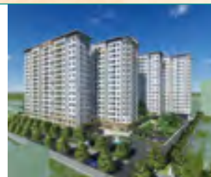
TDH - Phuoc Thinh Duc Apartment Building (Dist.9) Land area: 14,680 m 2 Ongoing
