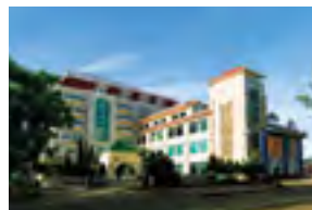
La Sapinette Hotel Dalat (TDH: 72%) Land area: 7,560 m 2 Completed in 2009 & transferred.
